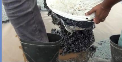
Pouring of Kavassu Rainsta Patch in Pothole gradually
