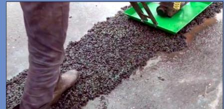
1st layer of compaction should be given through Plate Vibrators
