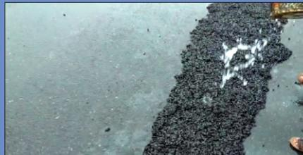
Clean water should be sprayed over laid road patch to cure it rapidly.
