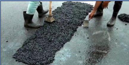
Manual Ramming should be done to prepare the surface for mechanical ramming
