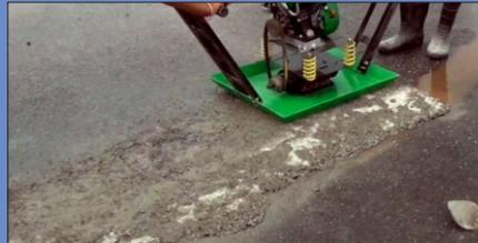
Again compaction through plate vibrator is done to fix all voids
