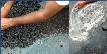
Filling of depressions and afterward powder additive should be sprayed over patch
